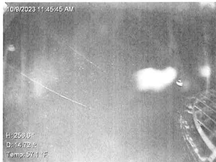
65) The bowl is covered with sediment that limited the amount of surface visible with the ROV.
