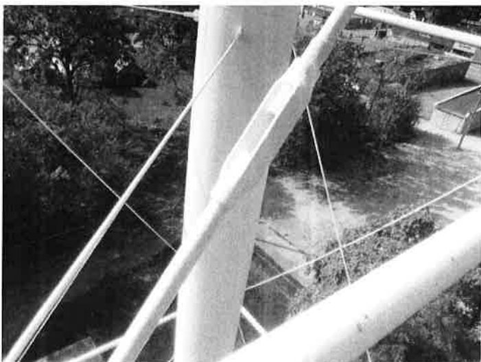
18) The sway rods are in good condition.
