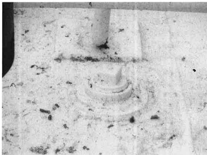
45) The roof rigging couplings are properly capped.
