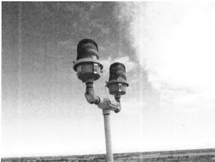
51) The double aviation light appears to be in good condition.
