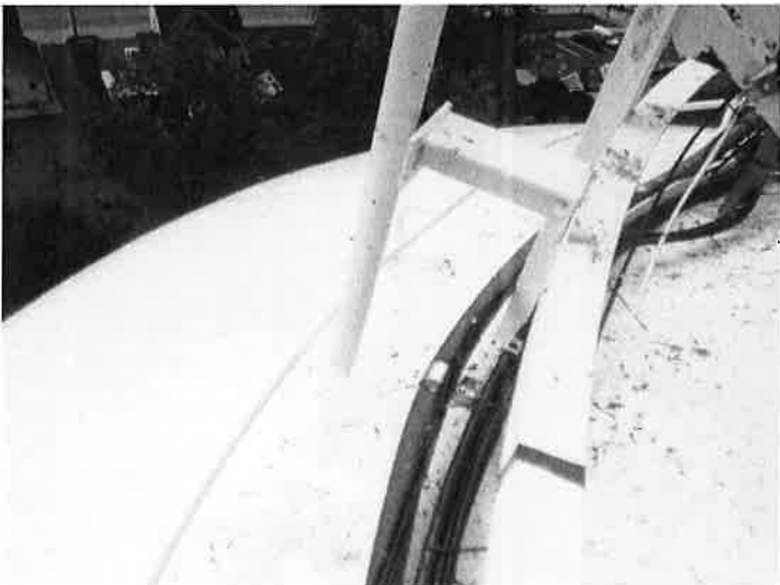
42) The roof coating is in fair condition overall.
