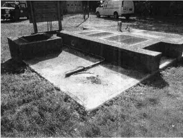
67) The metal hatch over the pit is in good condition.
